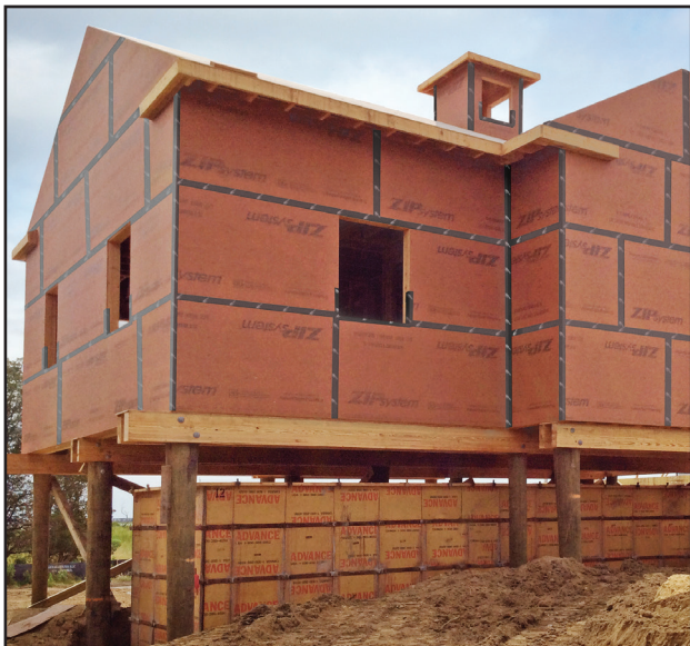
Left: Sunset Green Home used ZIP System® 1/2" sheathing, a structural 1 rated product.
